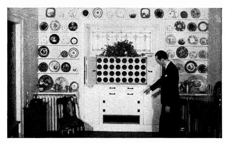
Fig. 15-13. A bank of thirty-two 6'' loudspeakers, provides wide angle high quality sound distribution.
