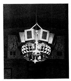
Fig. 22-27. A cluster of multicellular horns and LF speakers installed in Hershey Arena, Hershey, Pa. (Courtesy Altec Lansing)
