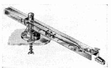
Fig. 10-17. Mechanical construction of the Pickering 190 Tone Arm.
