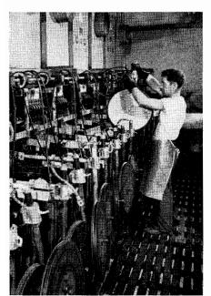
Fig. 27-3. Capper plating on a revolving hanger to insure even plating in a very active capper plating solution bath.
